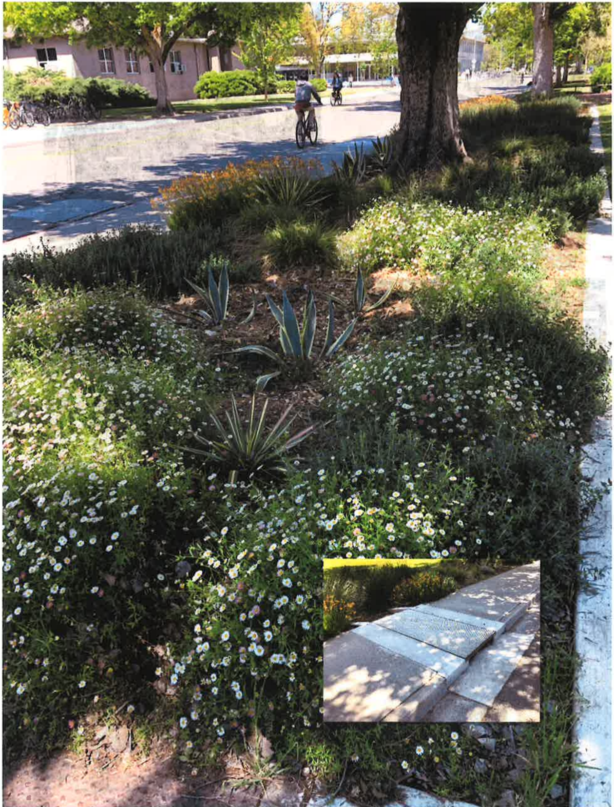
Figure 29 This is an example of a bioswale that receives water runoff from the street. The plants here can cleanse the water as it percolates into the ground.
